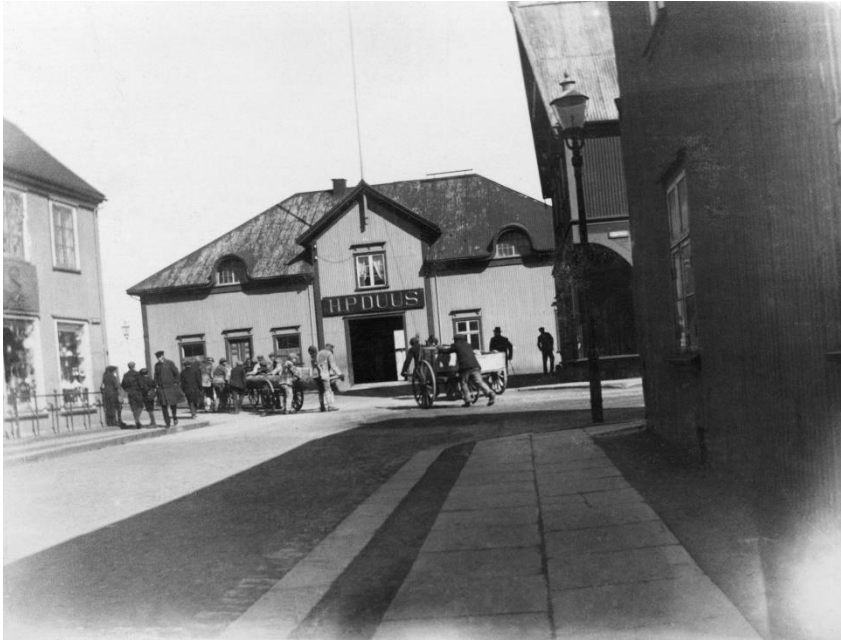
M25. Aðalstræti. View to the Vesturgata 2 . Street and constructions, around 1920 (LmsR, 2014 37 alb 004 3-1.jpg, Kristinn E. Magnússon)
