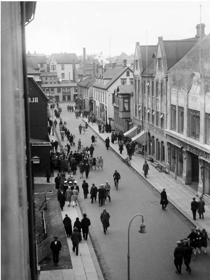
M26. Austurstræti. View to the Aðalstræti 6 and Grjótahverfi . Street (space division, road and pavements surfaces, lighting), 1926 (LmsR, ÓSG GLE 135.jpg, Óskar Gíslason (detail))
