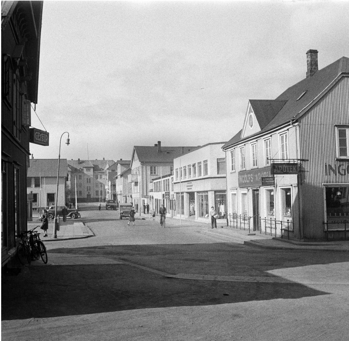
M36. Aðalstræti. View to the Hjálpræðisherinn . Street, building edges and constructions (right: Aðalstræti 2, 4, 6 and 8 ; left: Hafnarstræti 1 , Steindór Einarsson's taxi parking lot, Hótel Íslandsplan parking lot and Aðalstræti 7 ), 1948 (LmsR, LOG 007 4-1.jpg, Sigurhans Vignir)
