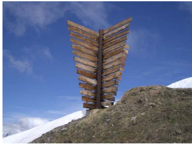
Fig. 12: Wind baffle, height 4.0m.
