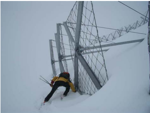
Fig. 11: “Ombrello”-structure fixed with one anchor.
