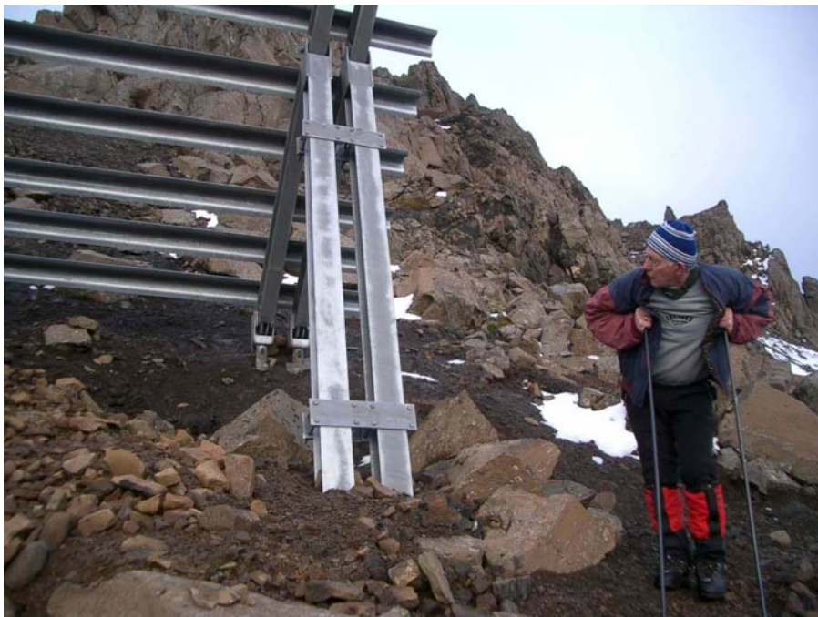
Fig. 8 : Reinforced end-structure in Gróuskardshnjúkur area, Siglufjörður.
